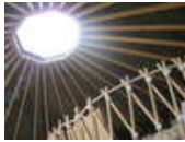
Building a new 20 foot gertee (Photos) by AlaskanTentLady
